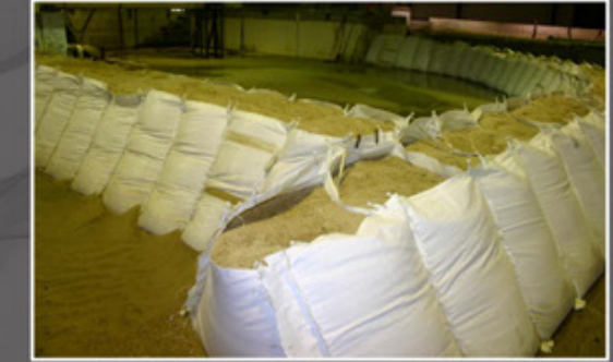
PermaShield™ system pre-test
