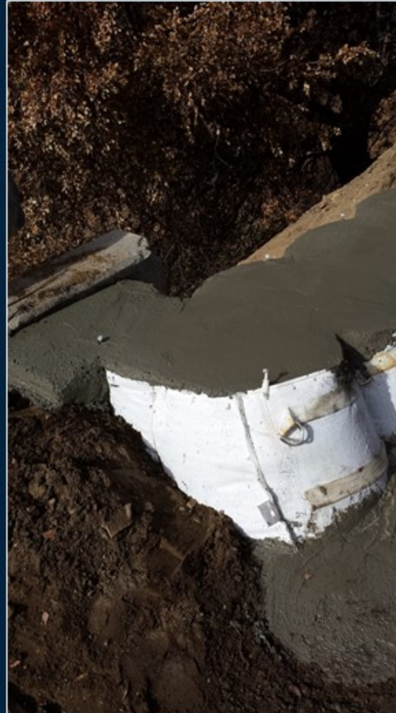
PermaShield™ system is turned to key into edge of existing headwall
