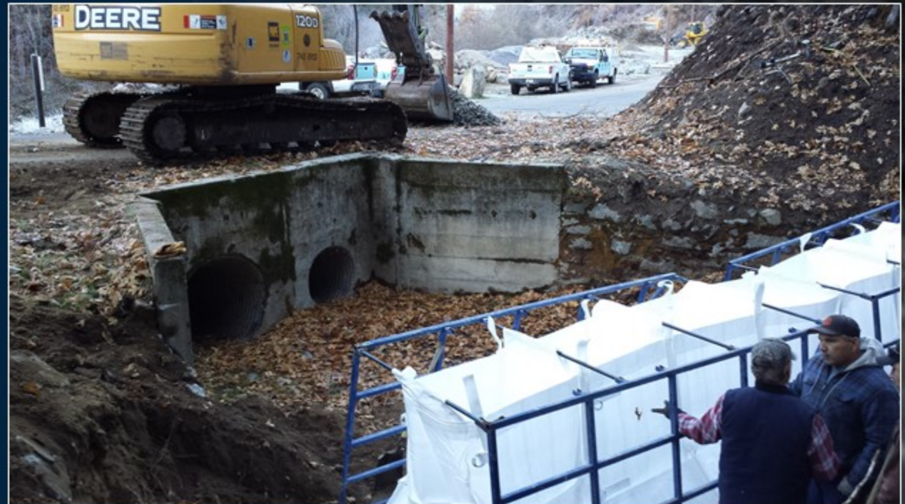
Culvert leading to Hetch Hetchy aqueduct
