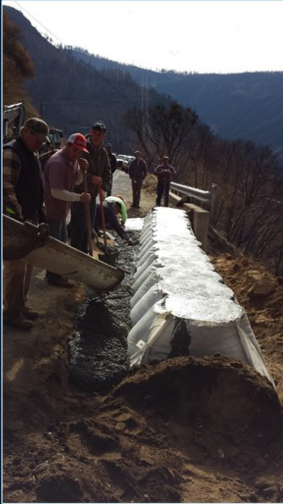
PermaShield™ filled with concrete and gutter being established
