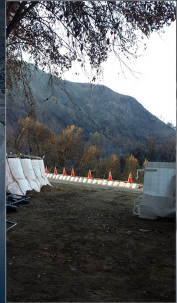
Looking at water diversion path to PermaShield™
