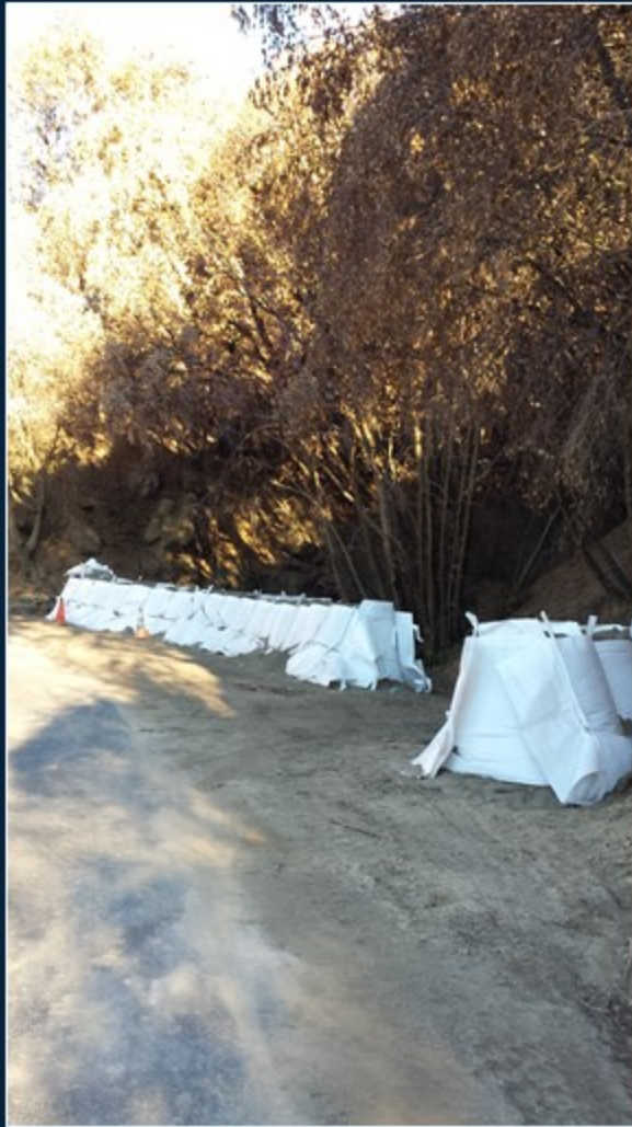
FlexiShield™ installed beneath runoff source
