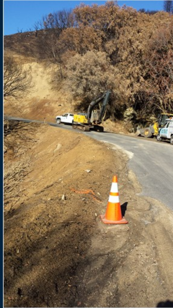
Road shoulder concern area
