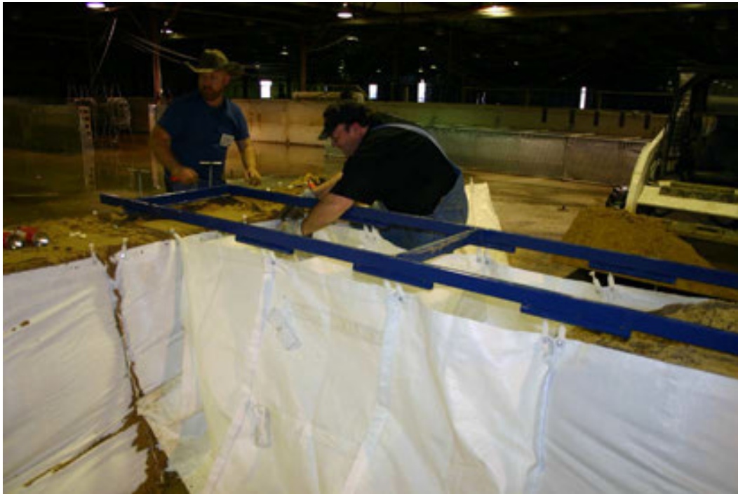
Figure 11. Portable frame used to hold bags open and in place where deployment trailer cannot be used.
