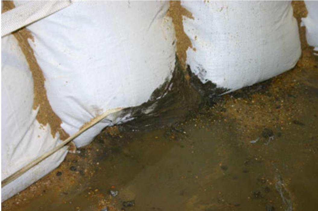
Figure 19. Concrete crack sealant applied to joint where seepage was high.
