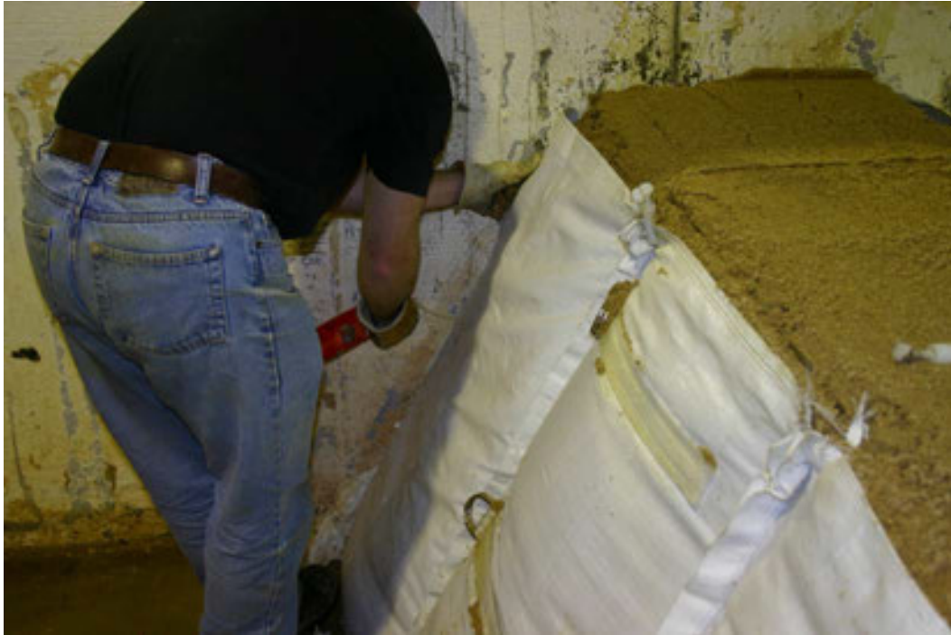
Figure 14. Expanding foam sealant completing the seal with the wingwall.
