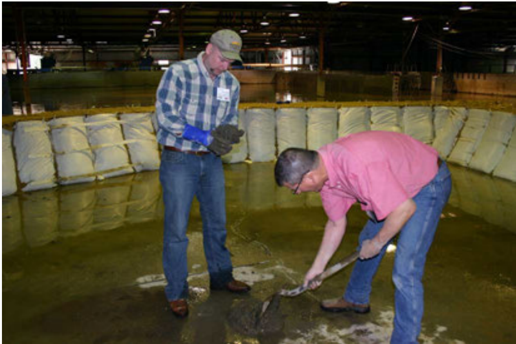
Figure 18. Concrete crack sealant being mixed in the test area.
