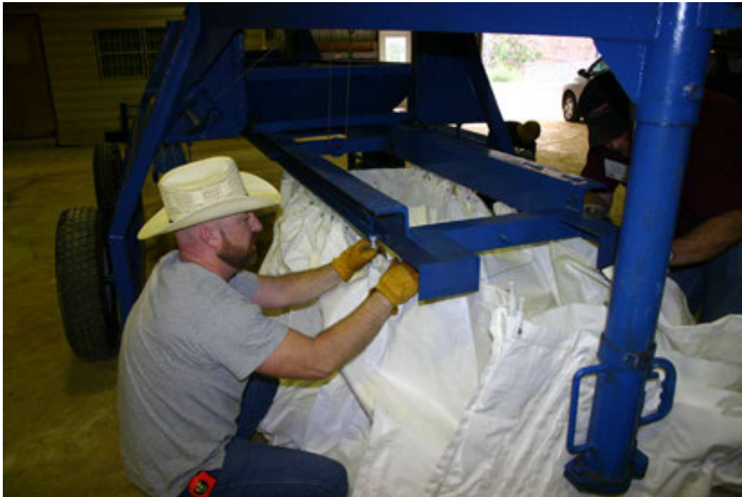
Figure 7. A 24-ft-long set of bags being loaded on the rails of the deployment trailer.
