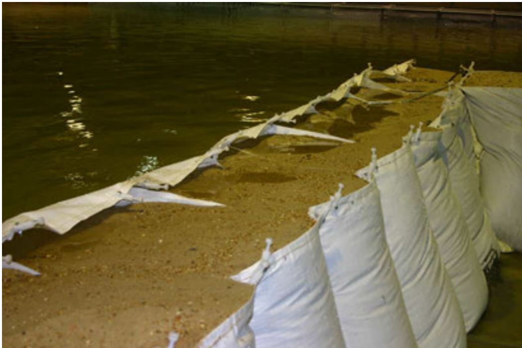
Figure 34. Wall "B" showing washout along outer wall of barrier at conclusion of test with medium waves at high water.
